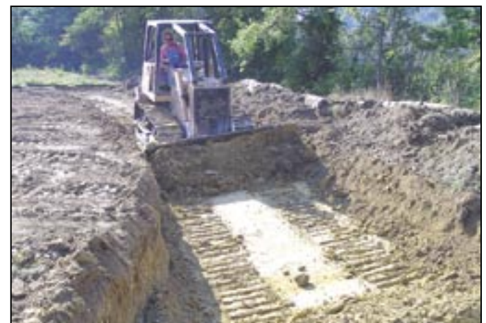
Core is located under the entire dam.
