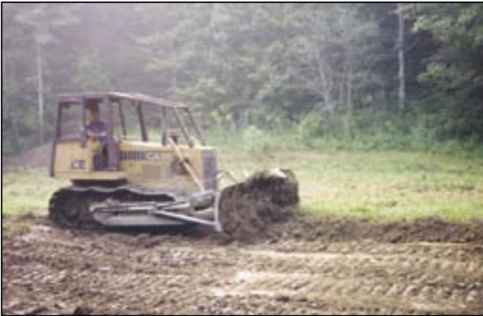
Remove and save topsoil.
