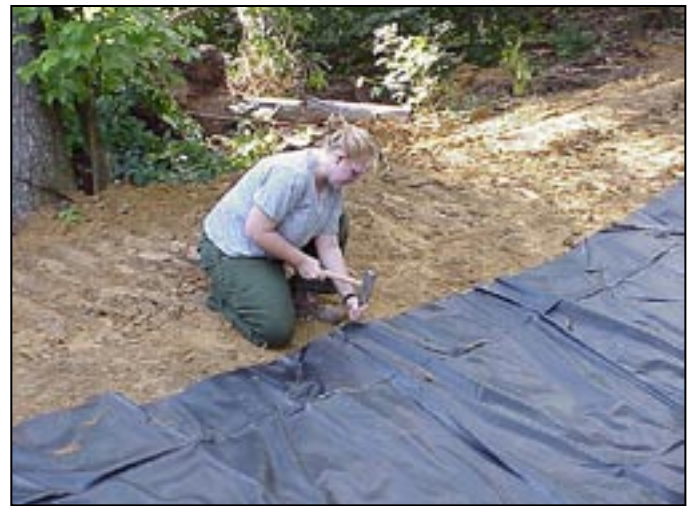
The liner is secured with stakes.
