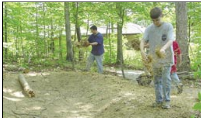
They seeded and mulched the exposed soil.
