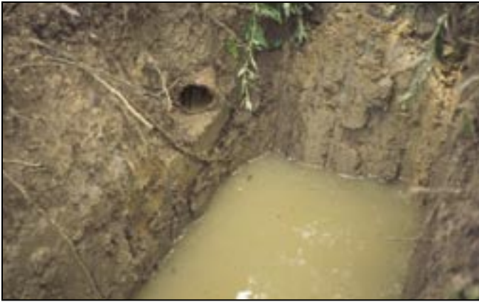
The core will crush buried drainage tiles.
