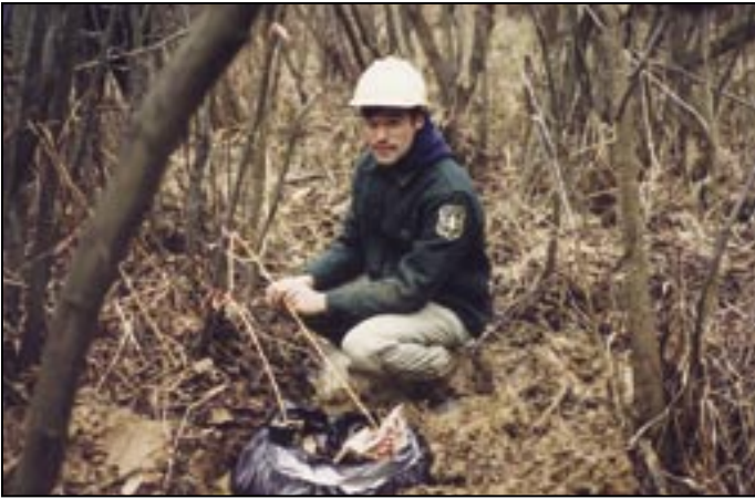
AN/FO is placed in a shallow hole.
