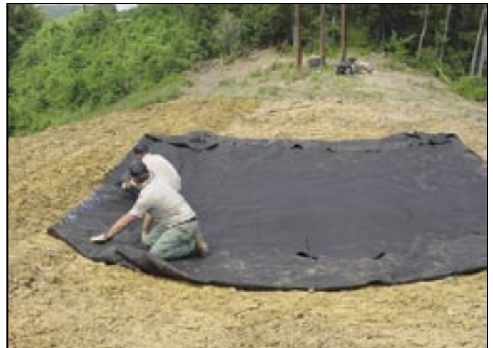
A liner is placed in the depression.
